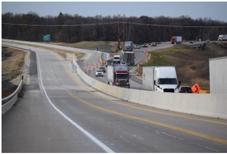
Hwy 14 Connection from 2-Lane to 4-Lane Looking West
