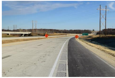
Hwy 14 Connection from 2-Lane to 4-Lane Looking East
